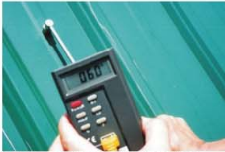
未施作COAT PC200前，屋頂板表面溫度 Surface temperature of the roof deck before application of COAT PC200
