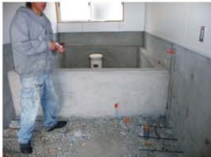
未施作伊凡特COAT PC200之前 Before application of COAT PC200
